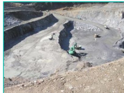
Koishwaragawa Dam construction (Blasting)
